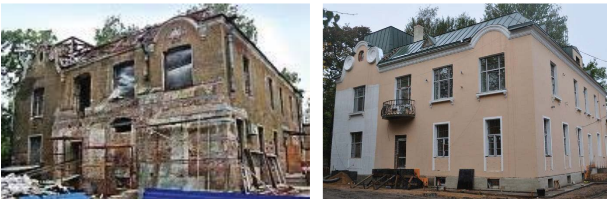
Fig. 5 – The reconstruction of the Technical office of the plant
